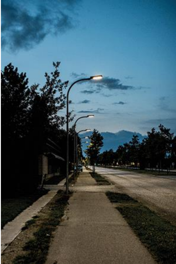
FIG. 1. Danish Outdoor Lighting Lab (DOLL) has over 9 km of test roads, pathways, and public areas and already has plans to expand. (Courtesy of Jeppe Carlsen/DOLL)
