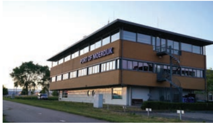
— Port of Moerdijk 2017
