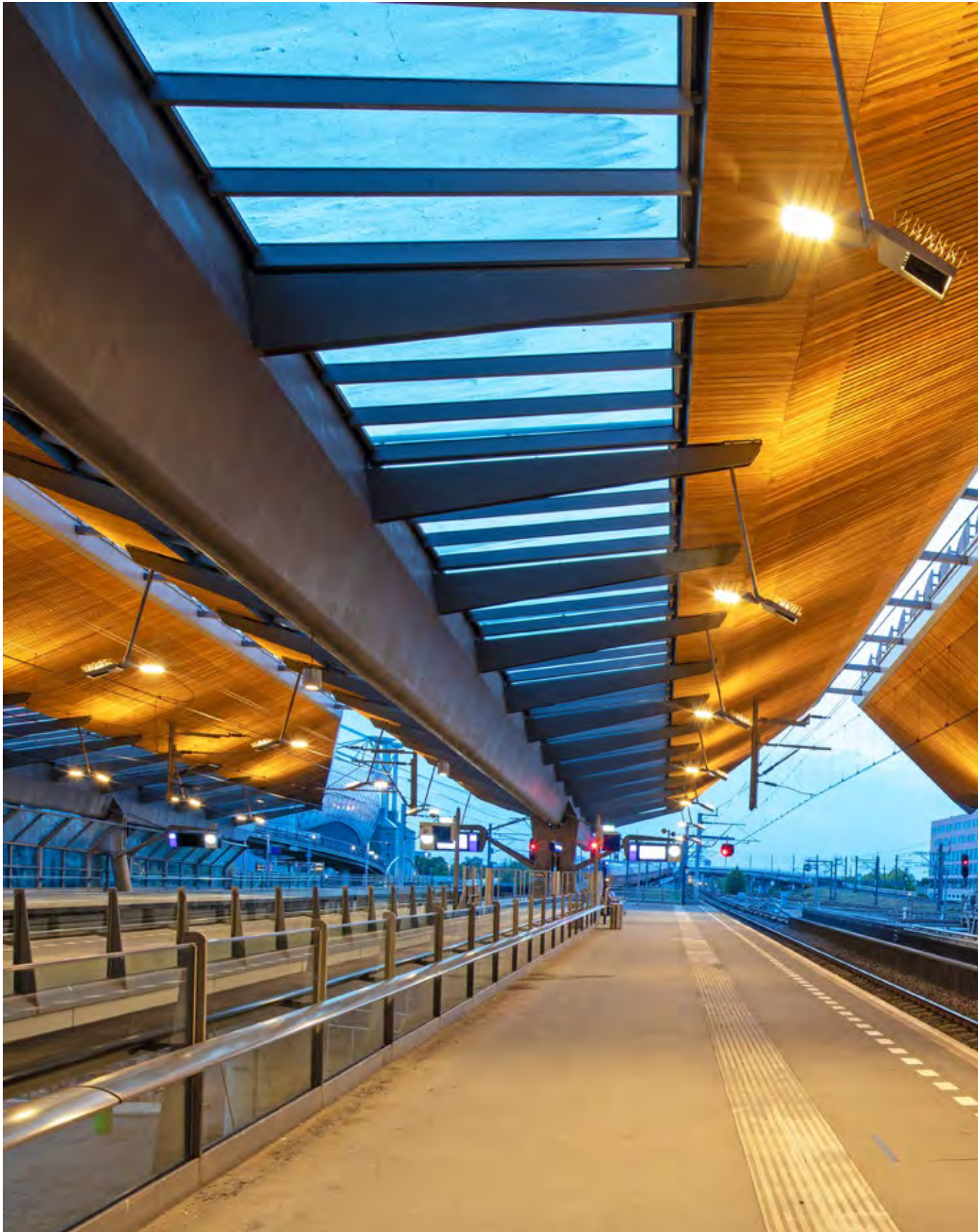
Up en downlighters station Amsterdam Bijlmer Arena na de led vervanging.
