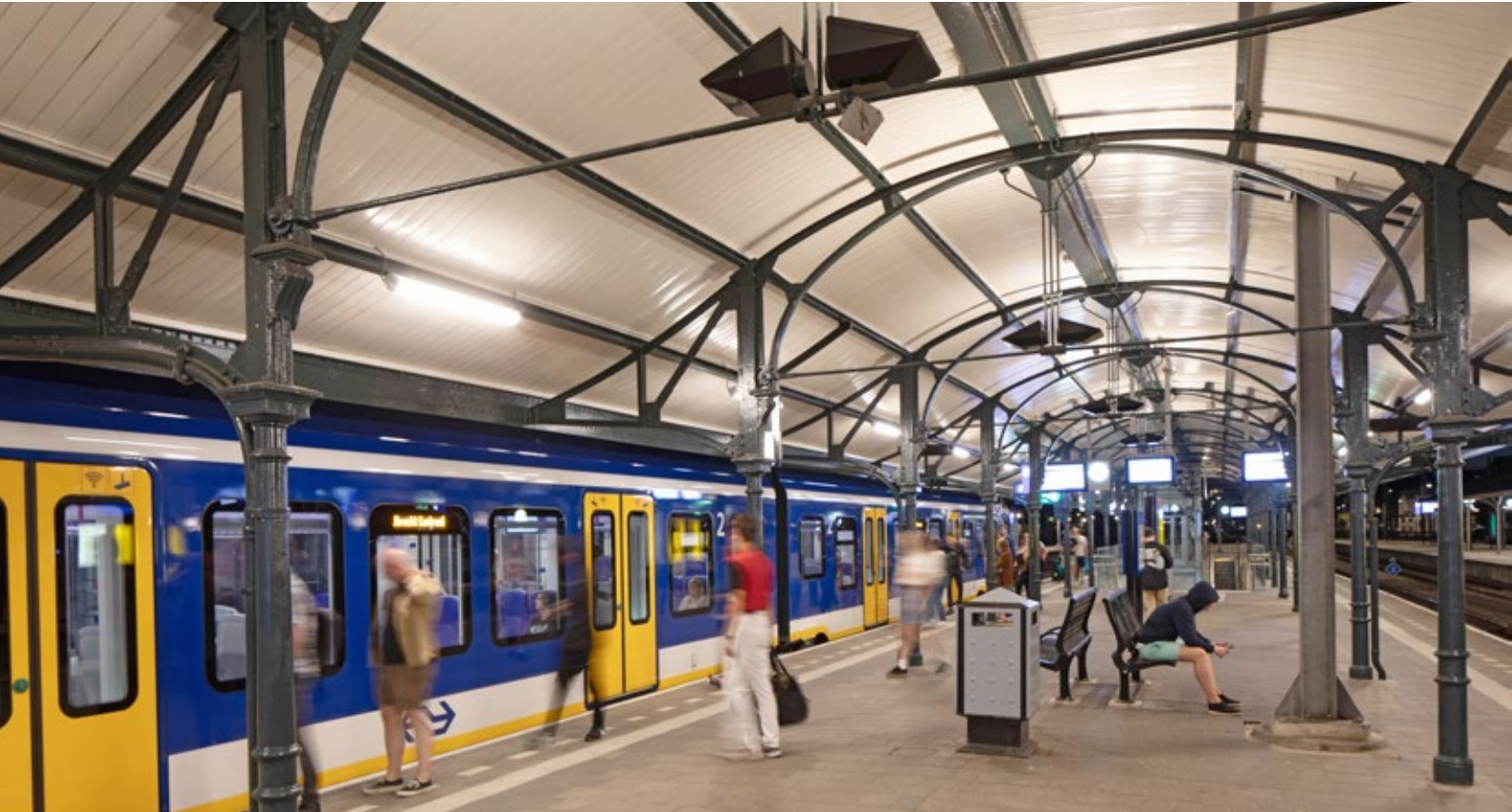
New uplighters under the canopy at Hilversum station with slanted pigeon-proof pane. The added fixtures above the tactile paving are visible on the sides of the canopy.
