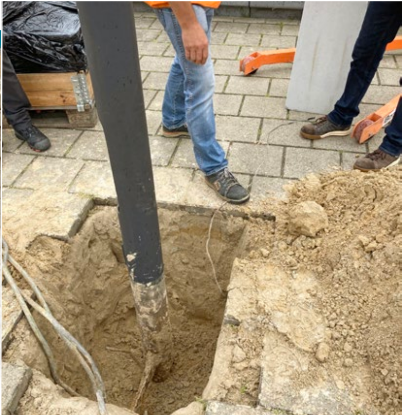
The old cable was dug up next to the old post.
