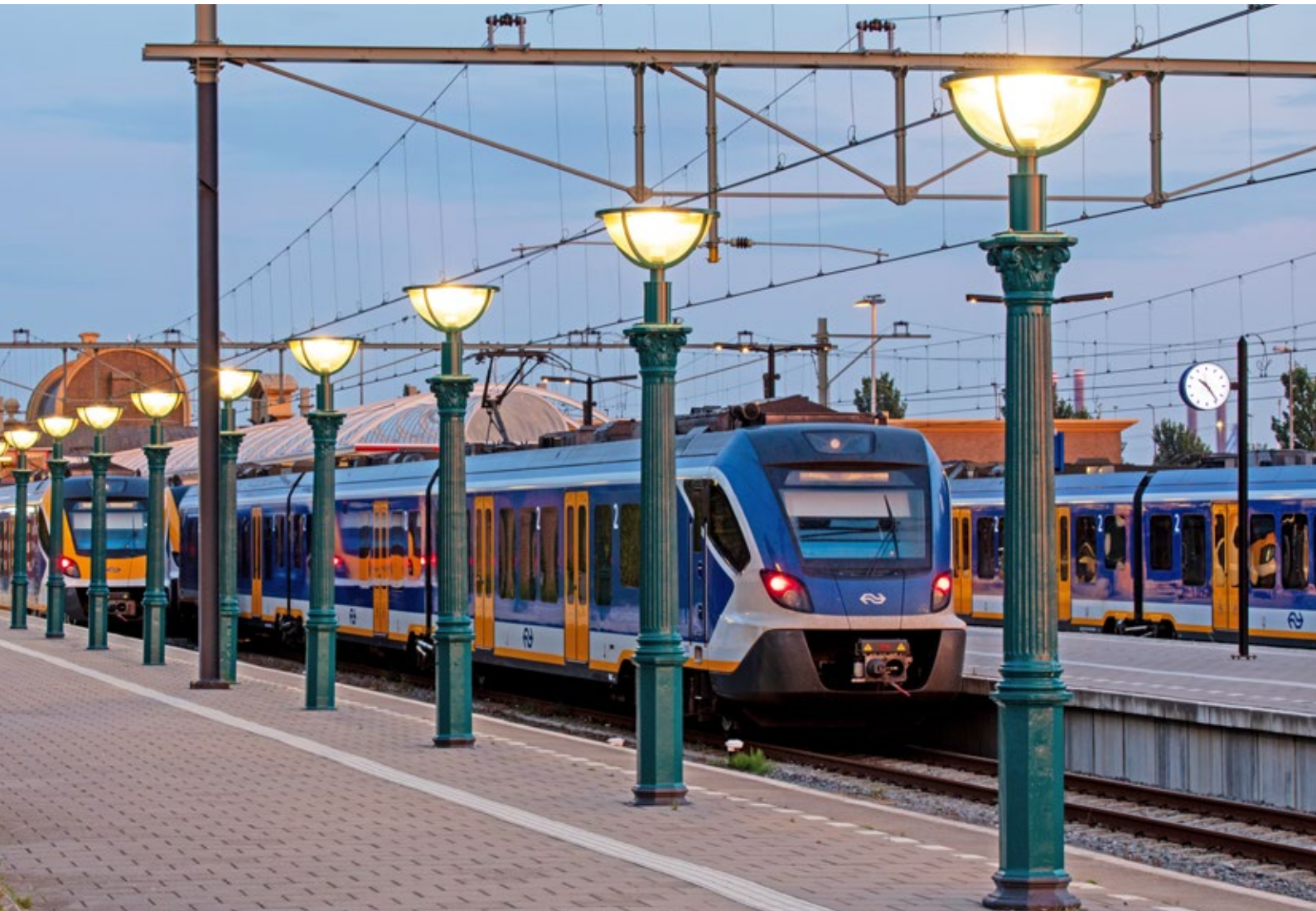
Historic cast iron lampposts at Vlissingen station fitted with custom LED fixtures and new transparent shades.
