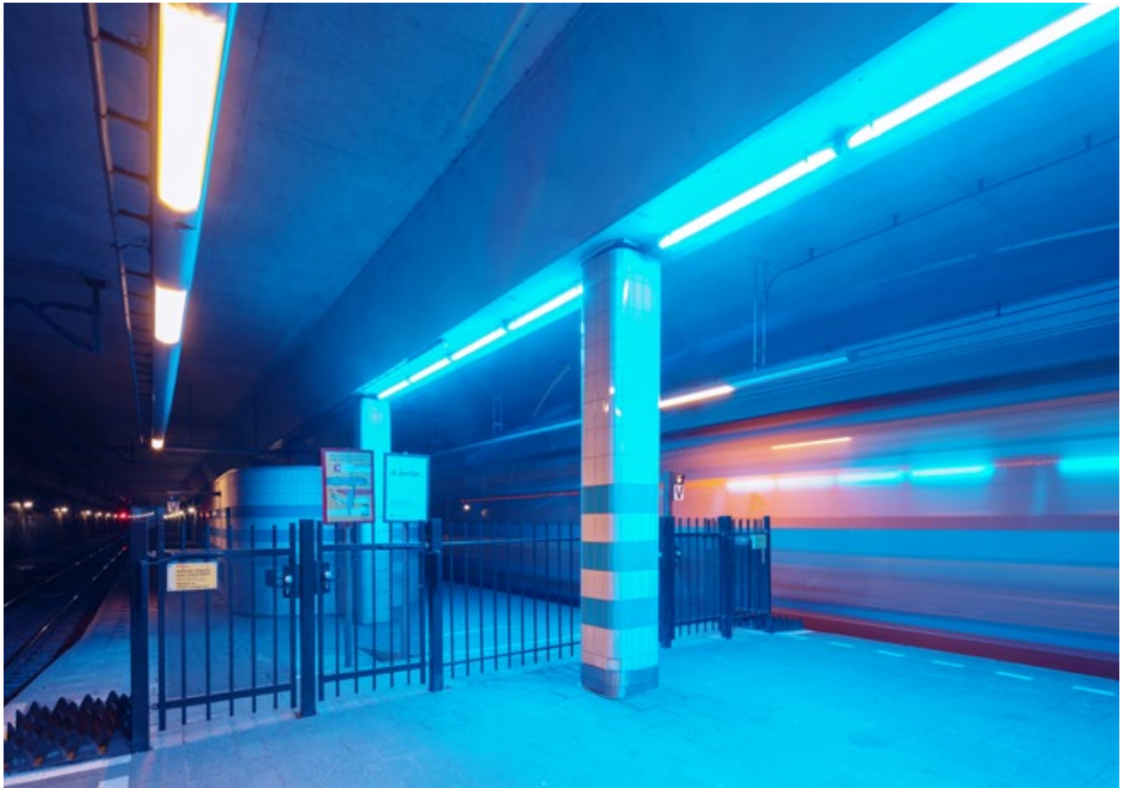
The end of the platform on the north side upon delivery in 2019, when the blue light turns on. Fences were installed to block off the end of the platform. The fence can be opened as an escape route, but was fitted with signs about the suicide prevention line 0800-0113.
