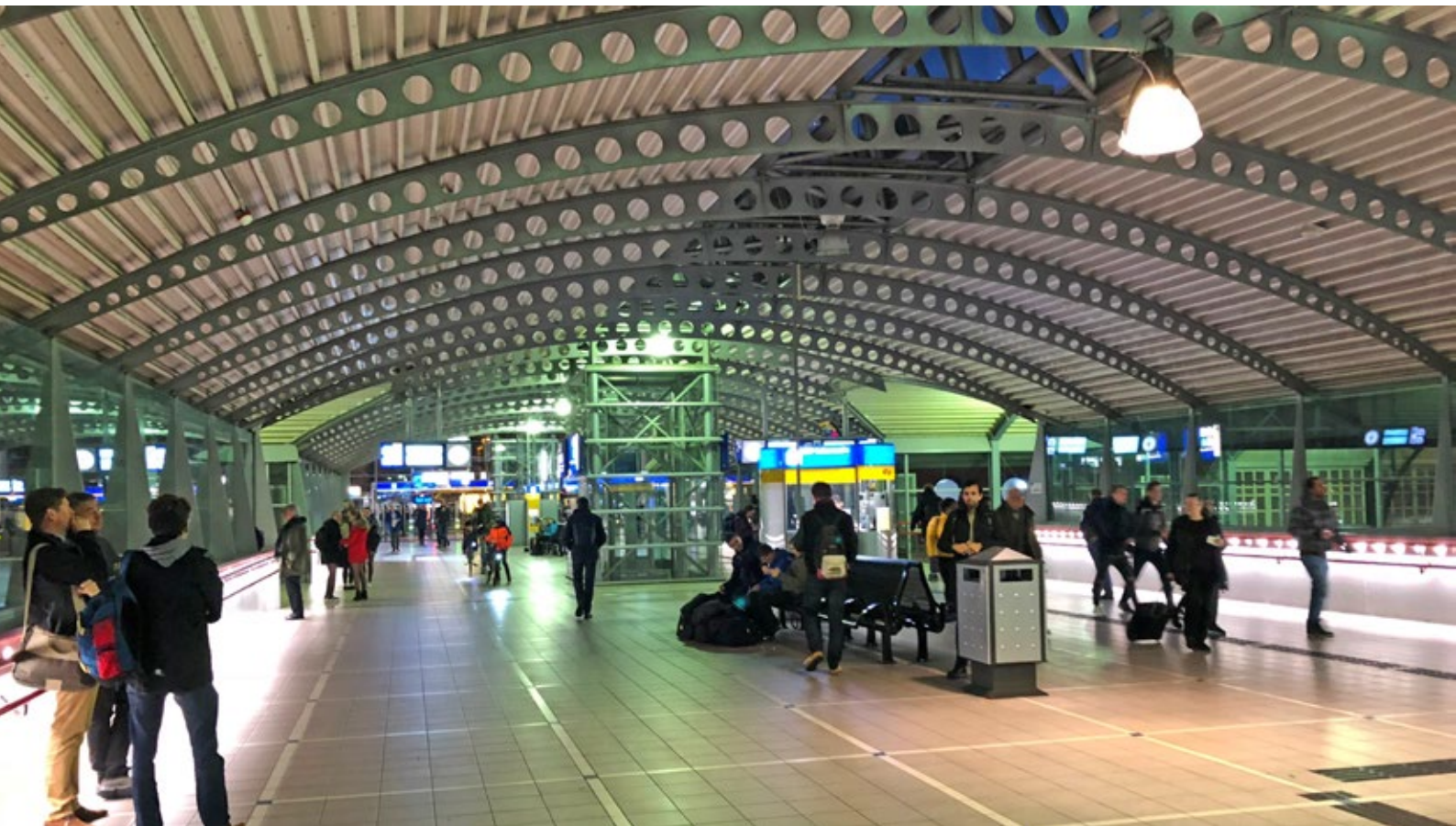
The test lighting setup at Amersfoort Centraal, with one LED chalice in warm white (2700K). This is the same colour as the line lighting along walls. In the background, an old mercury lamp with greenish light, with a colour saturation of just 20% ( R_a 20), while RLN00012 now demands 80%. At R_a 20, only 20% of the colours are discernible (pretty much just light and dark contrasts) and faces cannot be recognised. Difficulty recognising faces makes people feel unsafe. At R_a 80, enough colour is visible to recognise faces.
