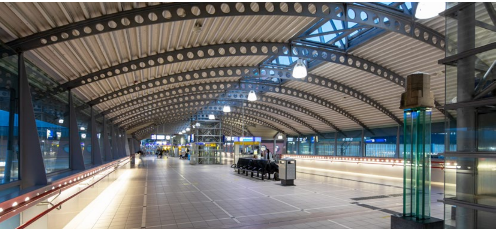
The indoor passage after replacement of all chalice fixtures in the evening situation, with warm white light. The floor is uniformly lit in one colour, which has a calming effect. The optics aim more of the light upwards, making the roof look better with crisper colours.
