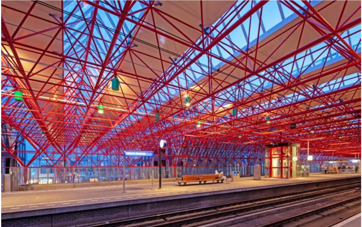
The present lighting situation. A slightly darker spot exists under the speaker (between the downlighters). Because the illuminance is much higher, it feels more comfortable. The canopy is more visible. We installed horizontally directed LED spotlights on top of the downlighters to illuminate the trussing from the inside out (i.e. away from the platform to avoid glare).
