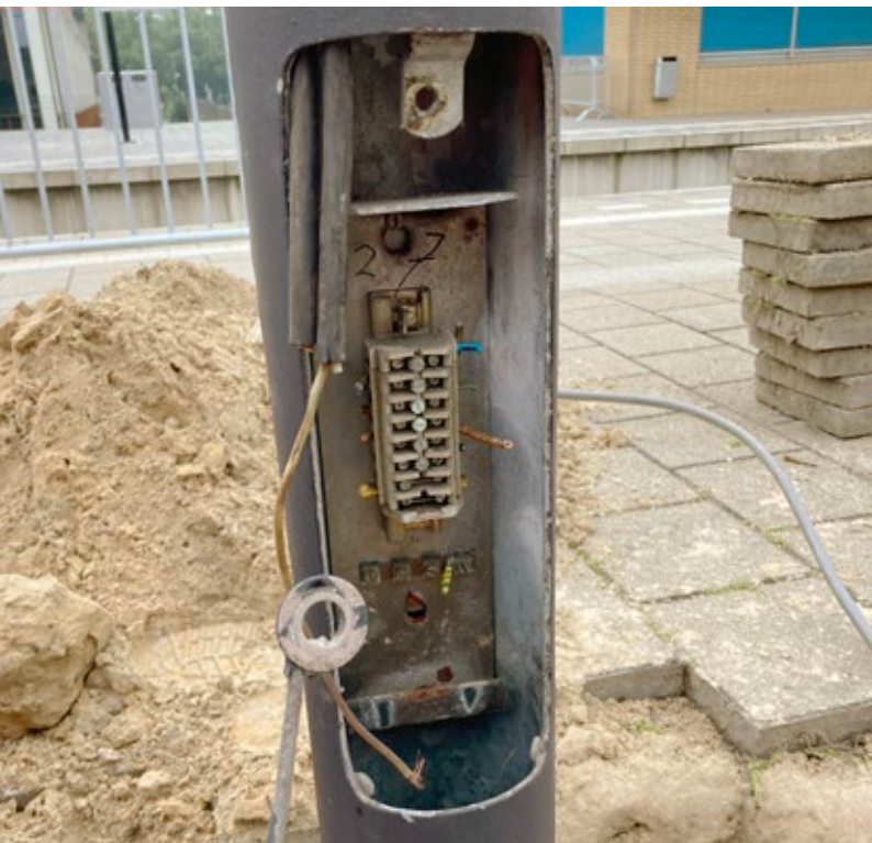
Removed the pole-rail connection (earth network between the old lampposts).
