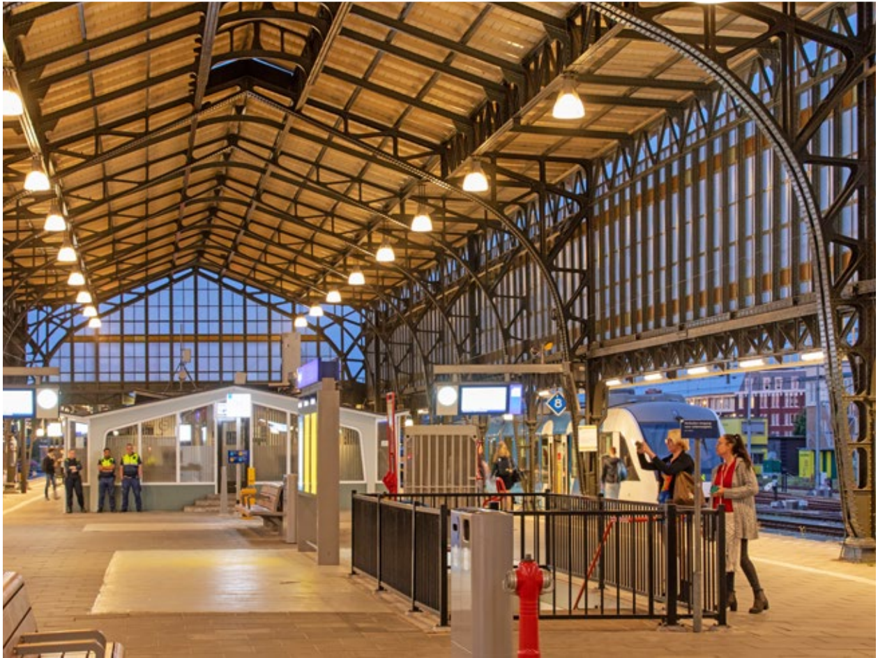
Monumental roof of Hengelo station. Existing chalice fixtures were fitted with new LED interiors (retrofit modules).
