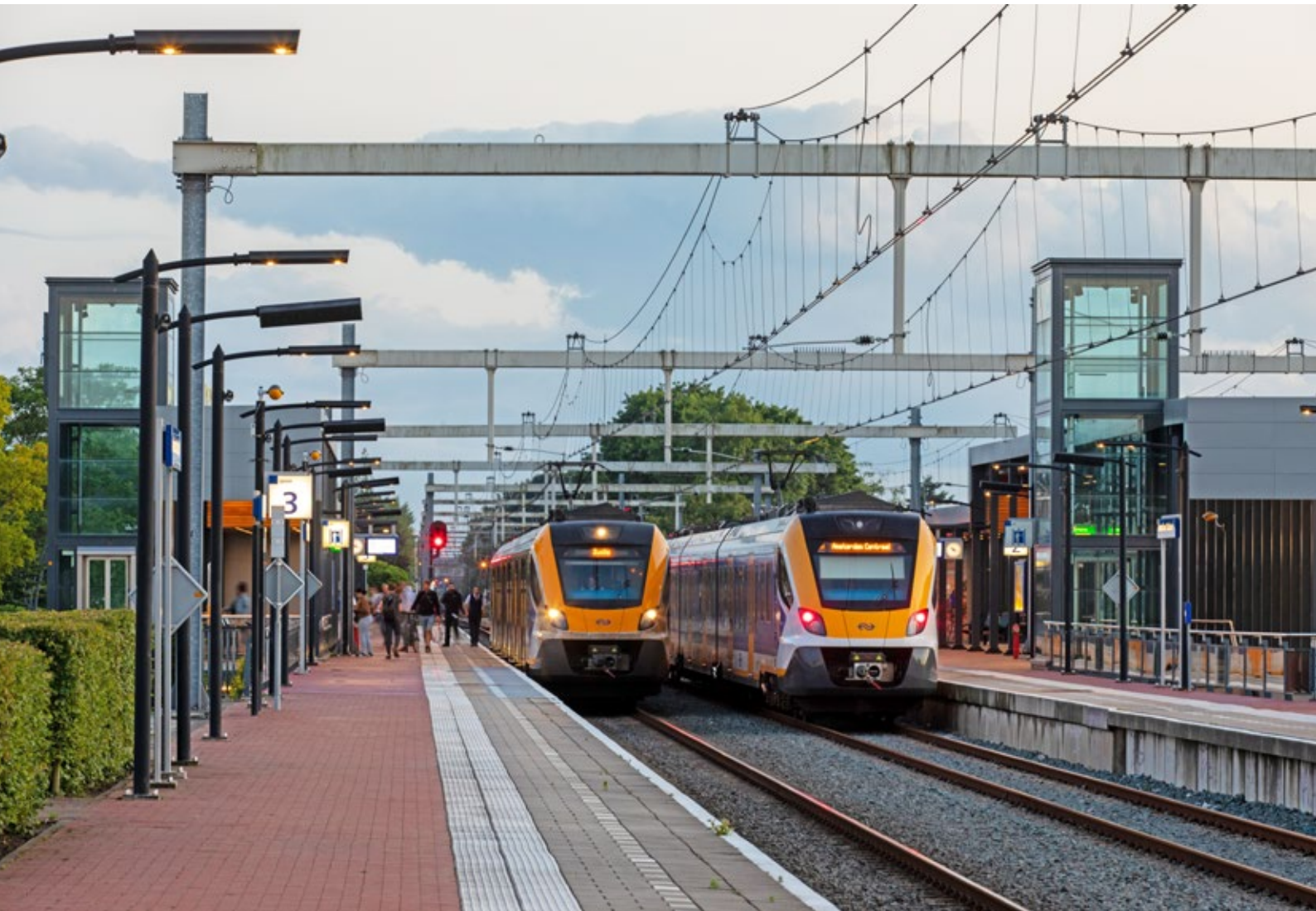
Vathorst station after the LED replacement. The separate speaker posts between the lampposts are very much visible. We want to avoid such a forest of posts with the Multi Purpose post (see chapter 18).
