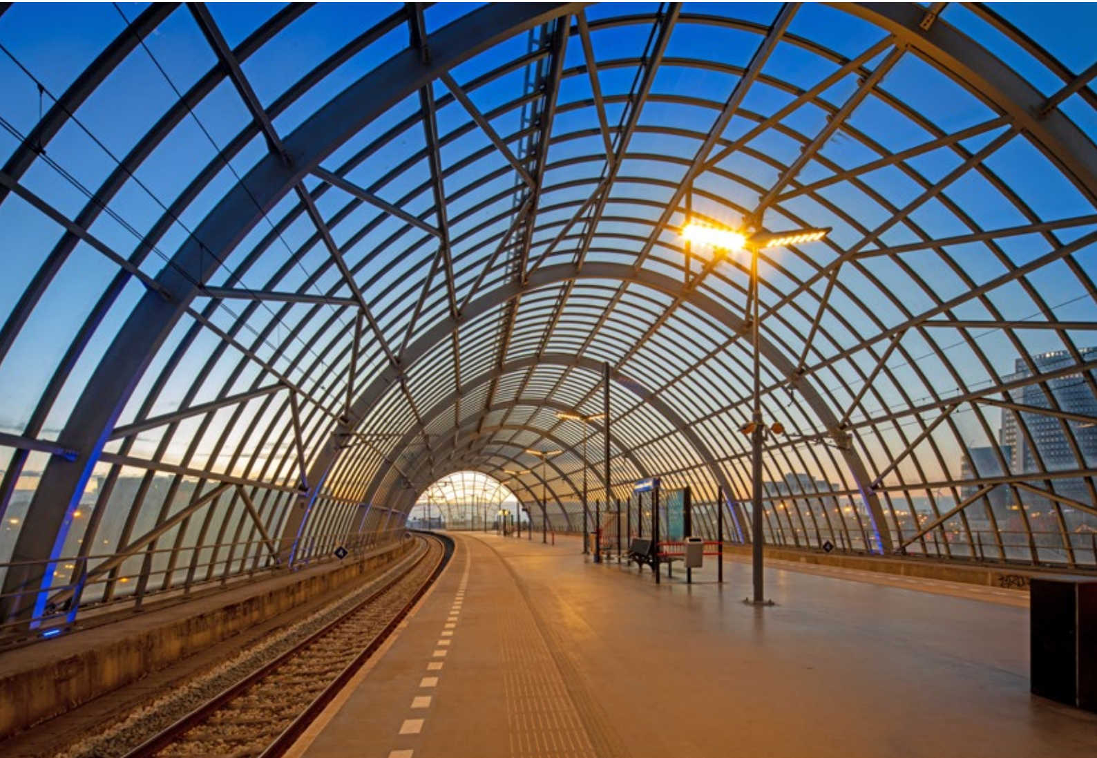
Amsterdam Sloterdijk station Hemboog. Not wanting to disturb the arches of the roof with fixtures, the architect opted for lampposts under the roof. To avoid glare, higher columns were applied than at regular platforms.
