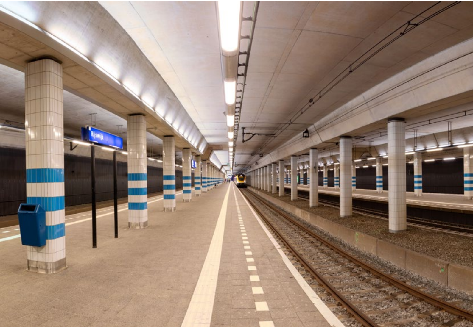
Uplighters cool white and downlighters warm white at the two central platforms at Rijswijk station.
