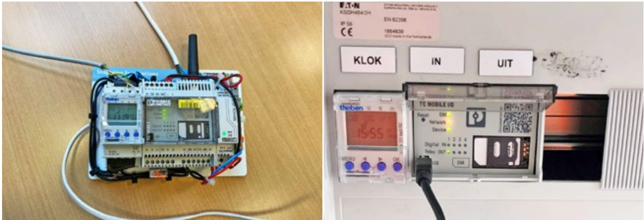
On the left, the test setup of GSM relay and timer. On the right, the built-in relay and timer at Arnhem Velperpoort station.
