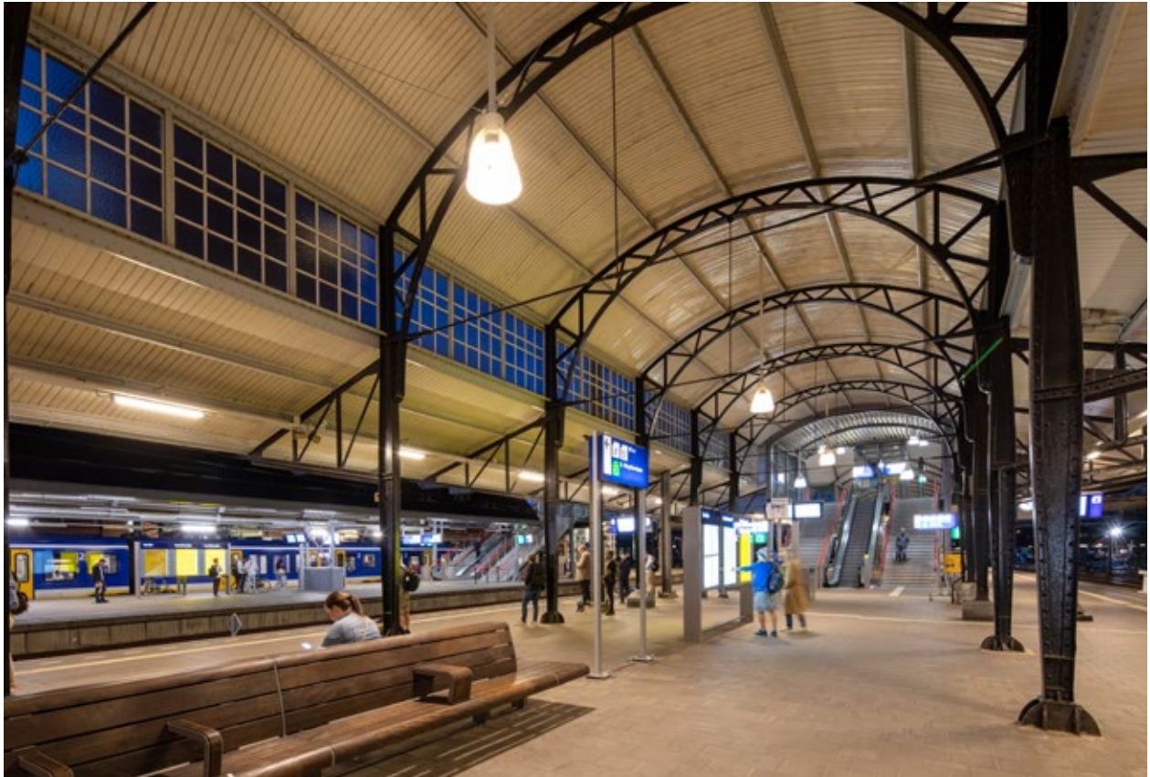
The platform canopy with new LED fixtures on pendants in the centre of the canopy and new LED strips (light colour 3000K) above the tactile paving under the flanks of the canopy.
