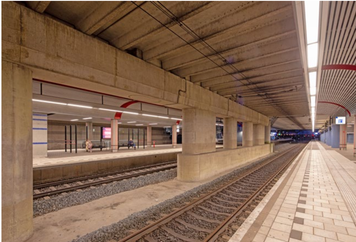
The fully enclosed platforms at Amsterdam Sloterdijk station with 200 lux in the evening after the LED replacement.
