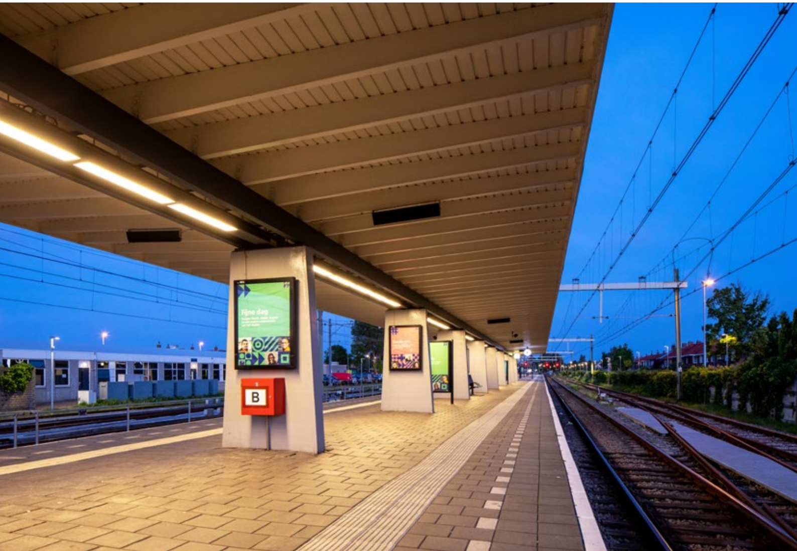
The sleek canopy at Den Helder station. Cables, ducts and pipes were concealed in the central girder (custom fixture in the girder cleaned and fitted with tailor-made LED interior).
