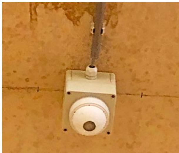
Sensors above the platform spaced every 30 metres
