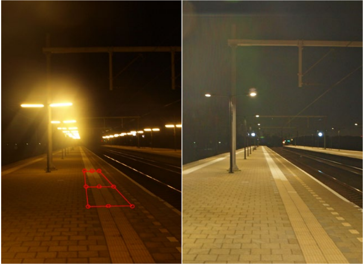
Voorschoten station, fluorescent on the left and LED on the right The 9 measuring points in red
