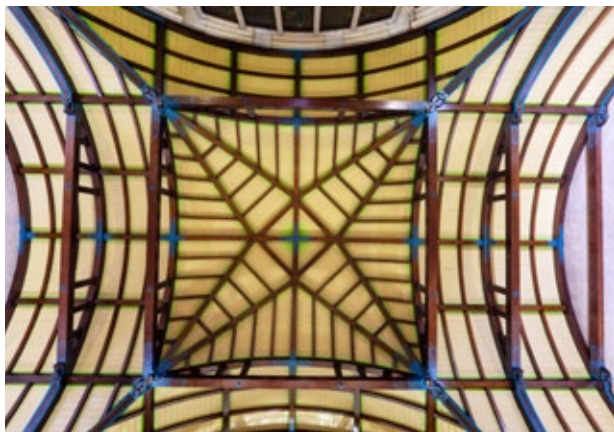
Roof construction of the train hall.
