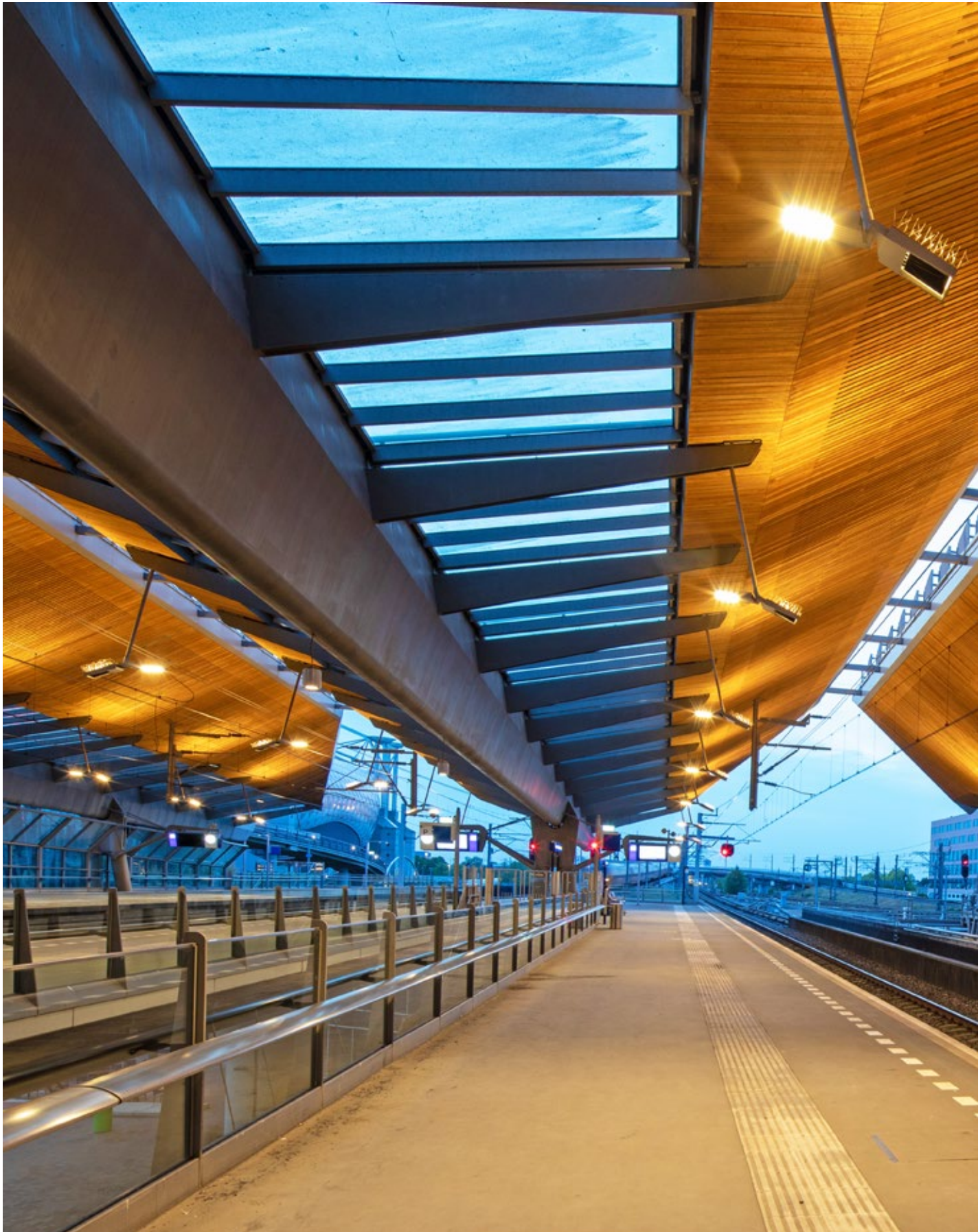
Up and down lighters Amsterdam Bijlmer Arena station after the LED replacement.
