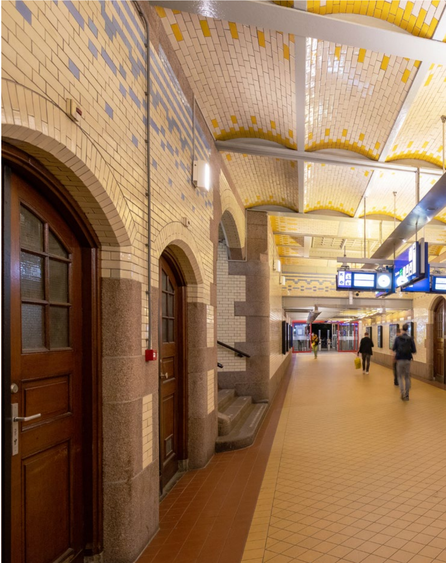
Indirect LED lighting in the passenger tunnel makes the remarkable masonry and tiles nicely visible (the lighting had already been replaced with LED).
