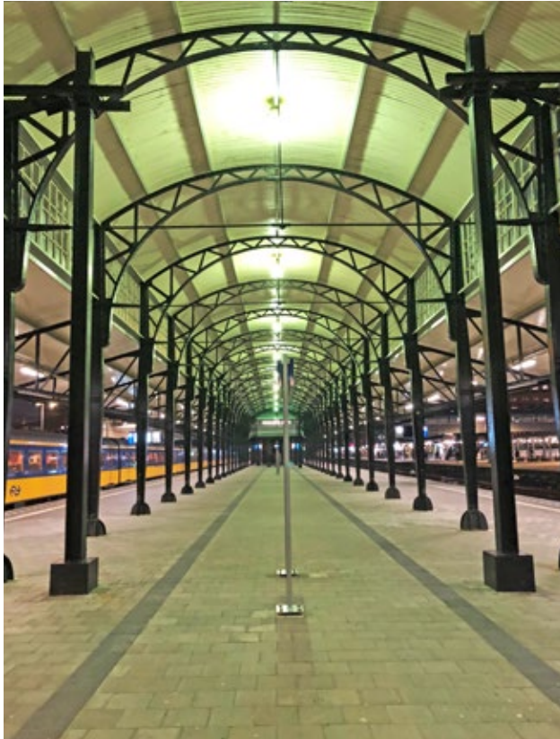
The canopy at Amersfoort Centraal with the old mercury lamps. The chalicees match the architecture, but give off a greenish light and were installed too close to the canopy. As a result, the canopy is lit in spots.
