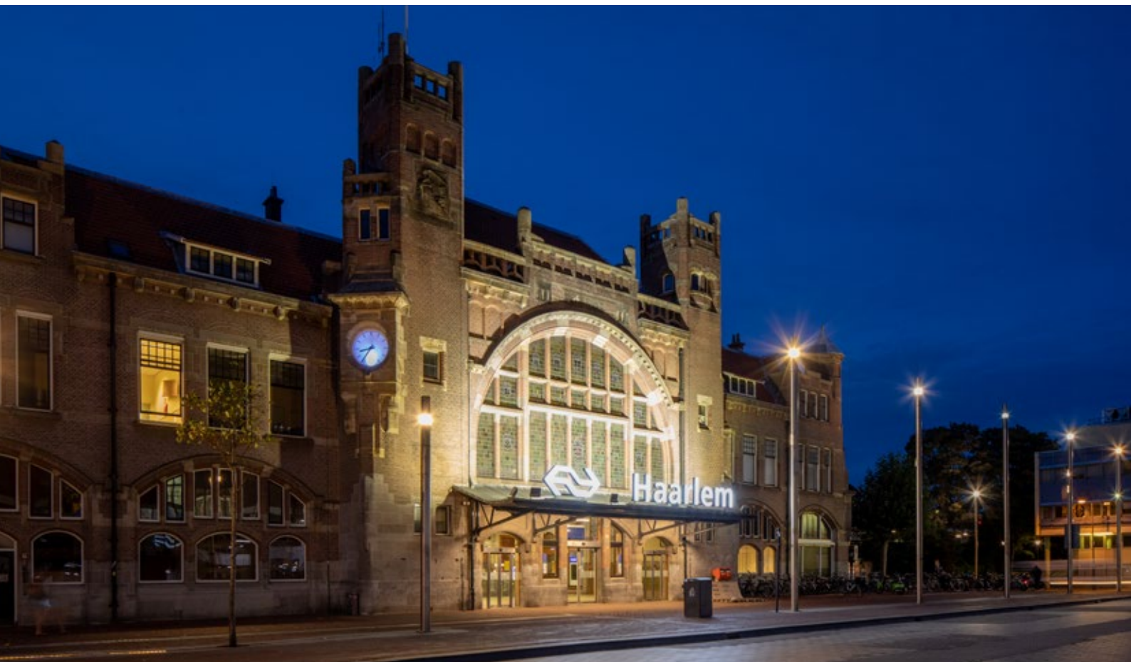
Entrance to the entrance hall already fitted with new LED lighting.
