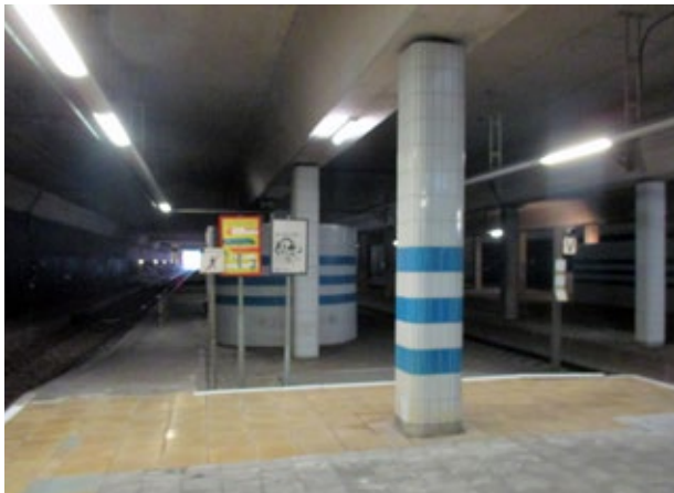
Rijswijk station in 2017, the end of the platform on the north side. Travellers were able to walk into the tunnel at the end of the platform using a ramp.
