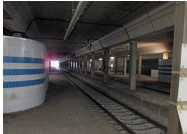
The end of the platform, right. Though daylight can be seen during the day, it turns into a gloomy place in the evening and at night.
