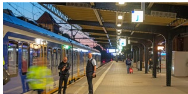
The Deventer platform after replacement.
