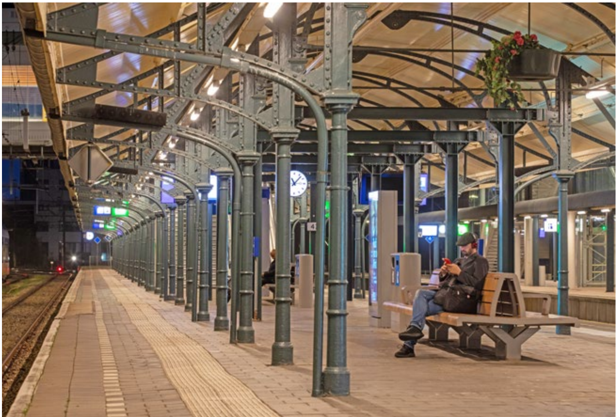
The monumental canopy with the new lighting
