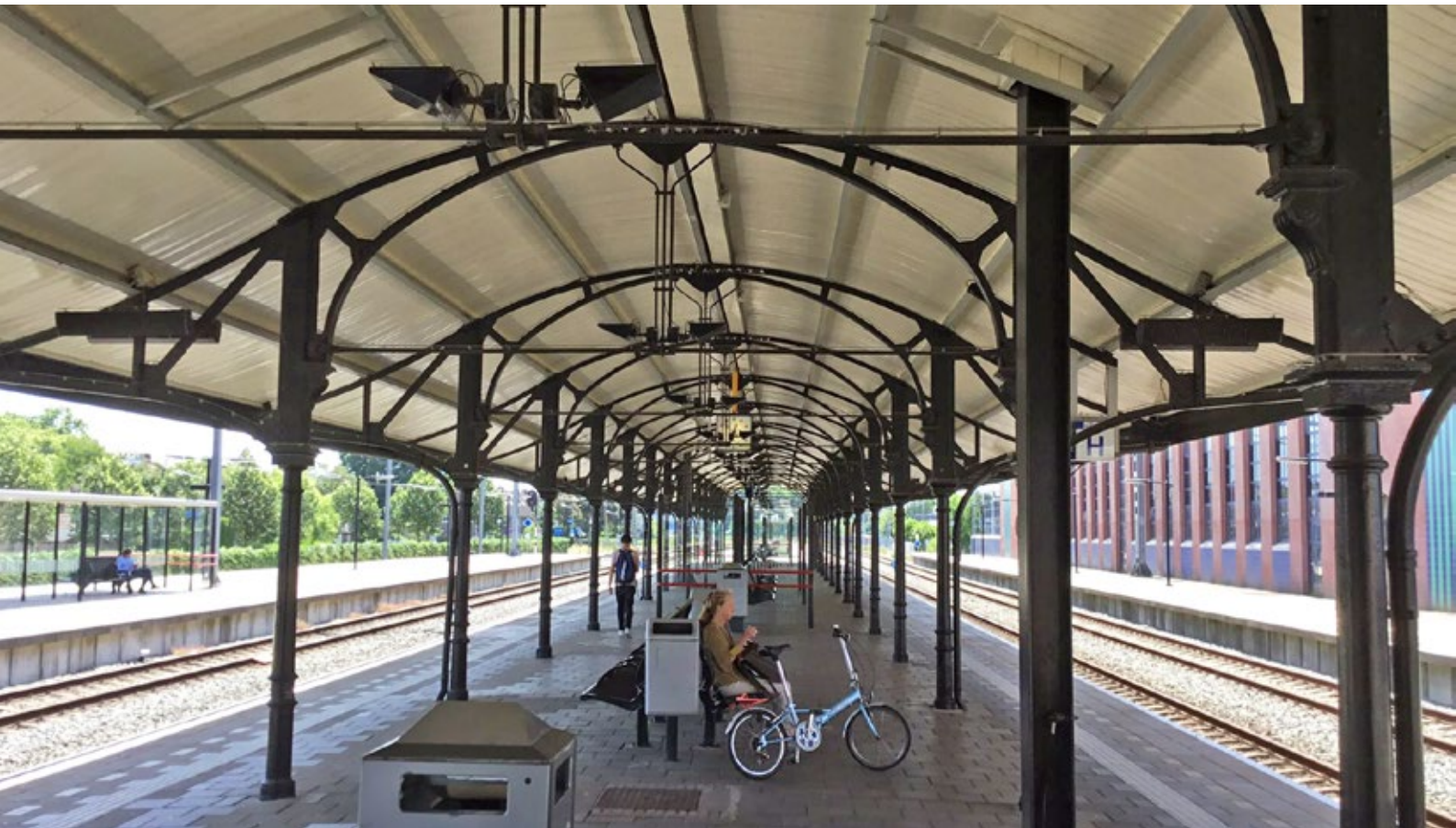
The old uplighters at Hilversum station with horizontal pane and anti-pigeon electric wire installation.
